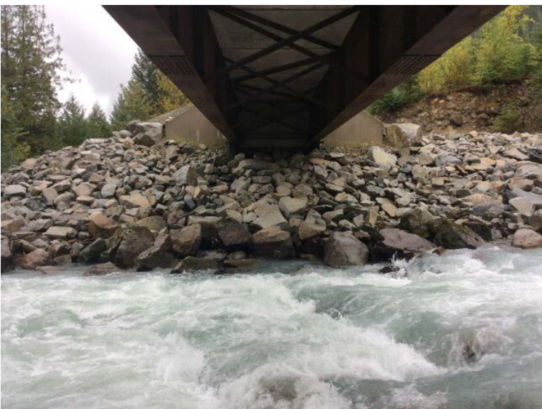
Right Bank Abutment when facing downstream
