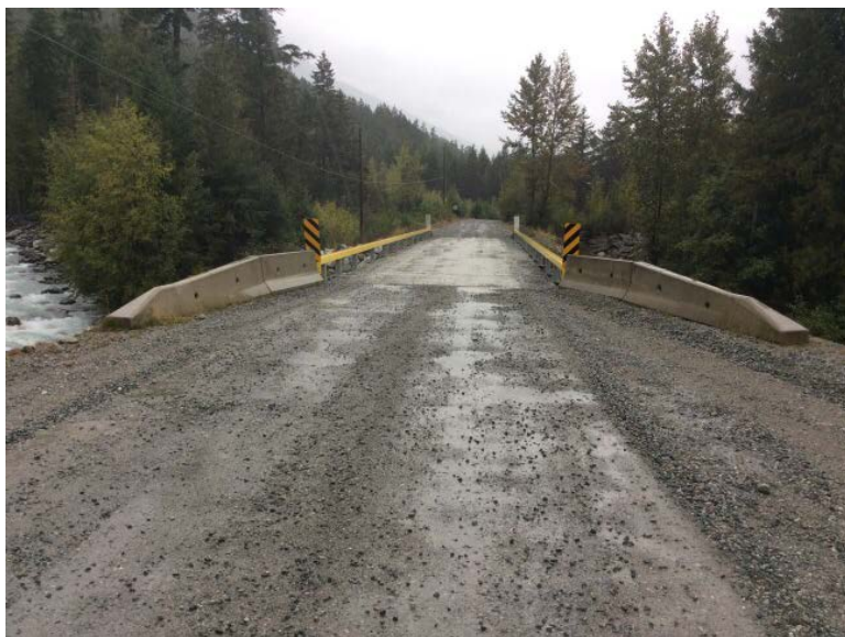
Approach from Right Bank when facing downstream
