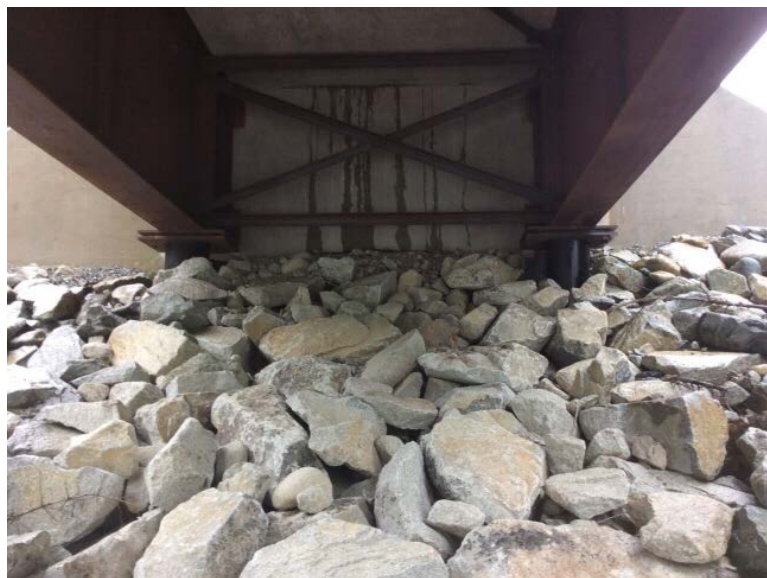
Left Bank Abutment when facing downstream
